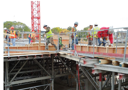
Construction Site and Temporary Office
